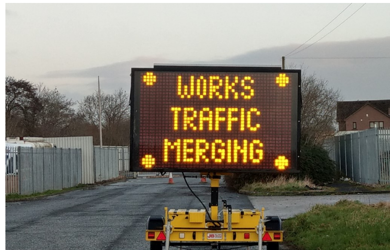
Mobile VMS on the A21 Kippington (Chevron, Costain) displaying Work's Egress activation message to passing motorists upstream from Site exit
